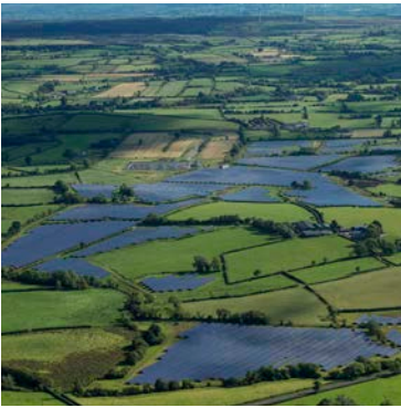
BayWa r.e. Project - Bann Road Solar Farm, Co. Antrim
