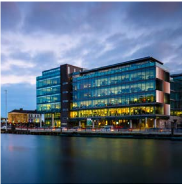
Johnson Controls, Global HQ, One Albert Quay, Cork
