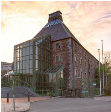
Heineken Ireland, Headquarters, Lady's Well Brewery, Cork
