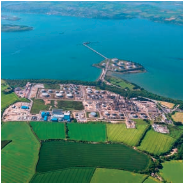
Irving Oil Whitegate Refinery, Cork
