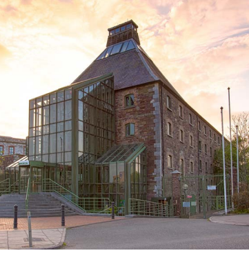
Heineken Ireland, Headquarters, Lady's Well Brewery, Cork
