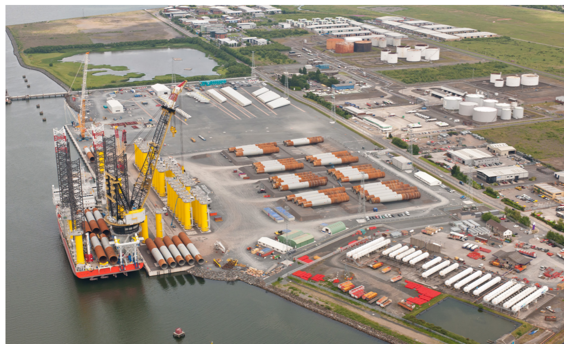
Figure 4.2. The development of a substantial number of offshore wind farms in the UK part of the Irish Sea, enabled Belfast Harbour to develop the first purpose-built installation and pre-assembly harbor in the UK and Ireland, at an investment of £50m in 2013. Initial turbine sizes were 2.3MW. The port remains an unrivalled facility in the Irish Sea with 480m of quay, 9.3m channel depth, and 50 acres of storage area. It was developed under a long-term agreement due to visibility of a large project pipeline (West of Duddon Sands 389MW; Burbo Bank Extension 232MW; Walney Extension 660MW). Belfast Harbour serves as a role-model for what can readily be achieved in Cork Harbour in support of offshore wind. Companies such as the Doyle Shipping Group are uniquely placed to transfer stevedoring expertise and offshore wind know-how from Belfast to Cork. Image source: DSG.
