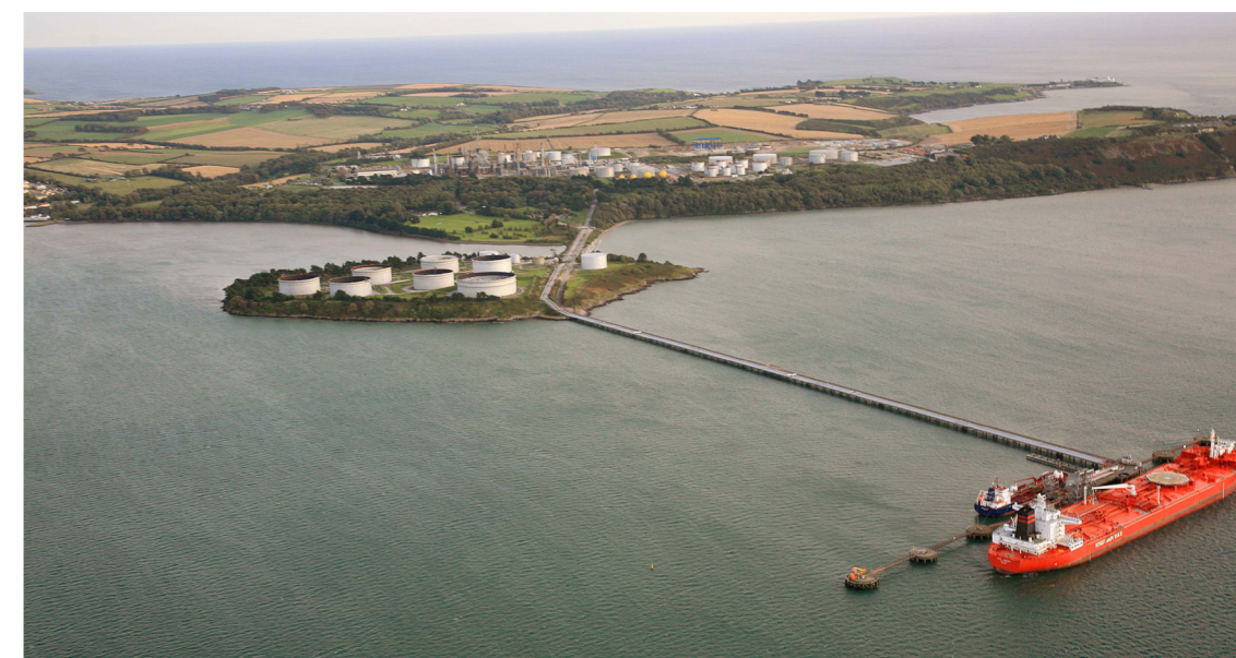
Figure 3.4. View looking east from Cork's 'Energy Quarter' in Lower Cork Harbour, including the oil refinery and the Bord Gáis Closed Circuit Gas Turbine (CCGT) Plant at Whitegate. Hydrogen from natural gas is consumed at scale in this industrial cluster. Green Hydrogen generated from electricity produced from floating wind, has the potential to support the decarbonisation of such industries, for example by providing dispatchable power through CCGTs. Image source: Port of Cork Company.
