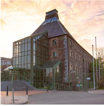
Heineken Ireland, Headquarters, Lady's Well Brewery, Cork
